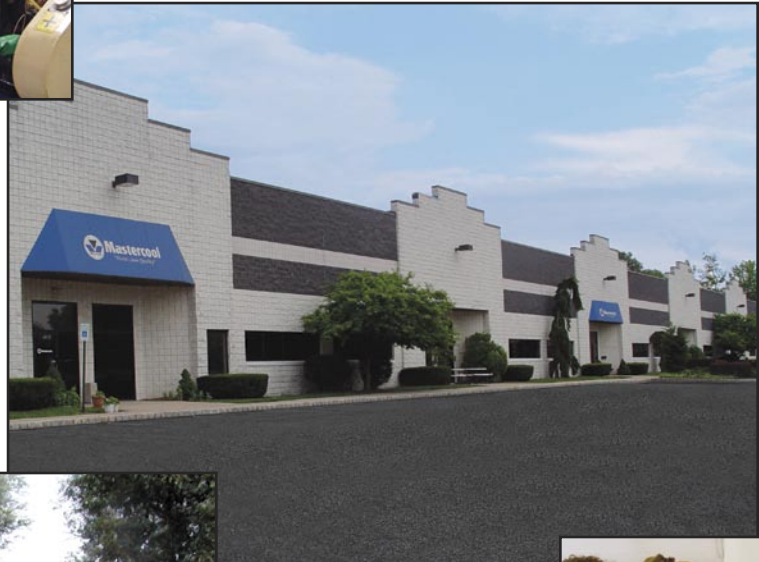
Corporate Office Manufacturing and USA Warehouse
